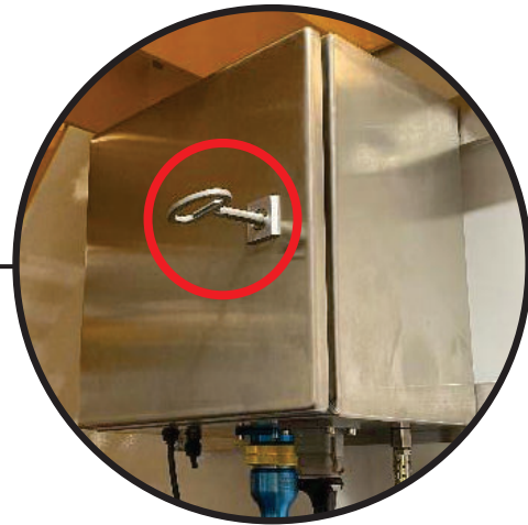
Figure 16. Control box key stored in the cab
